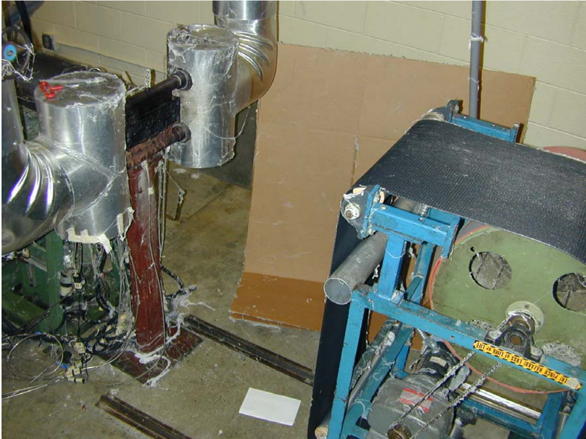
Figure 5.1-1: The TANDEC 6-inch pilot line (photo by Chris Eash)
