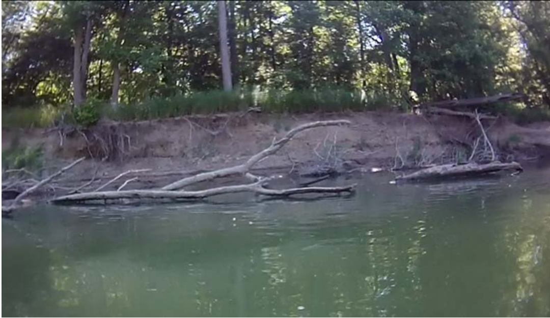
Figure 7.25. Driftwood River site with a low percentage of bank surface protection. This streambank location received a high bank erosion susceptibility rating, mBEHI score = 36.80.
