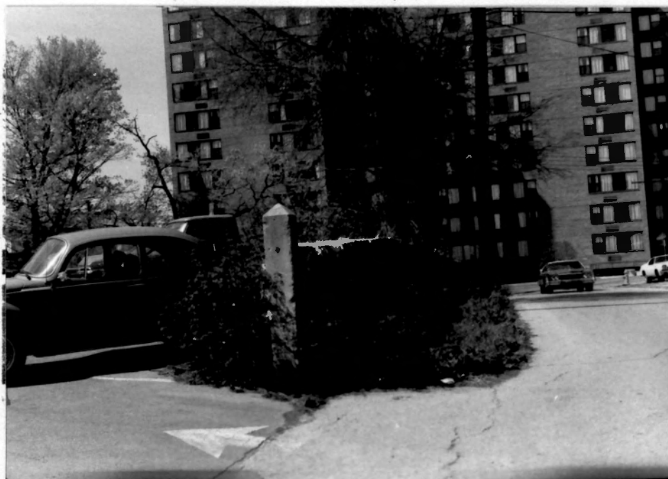
Figure 30. Impassable sidewalk on Hickey Place.
