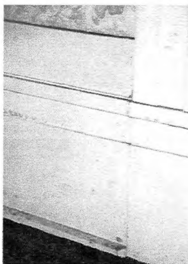
Figure 43. Baseboard molding Cannon-Stickley Home
