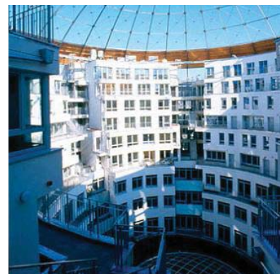
FIGURE 17. View into Gasometer C
