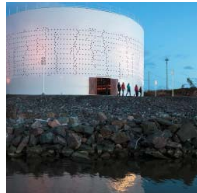
FIGURE 24. Exterior of Silo 468
