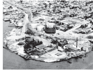
FIGURE 8. Decommissioned gas works plant
