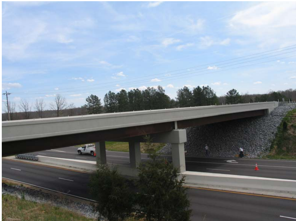
Figure 2: Photo of the DuPont Bridge
