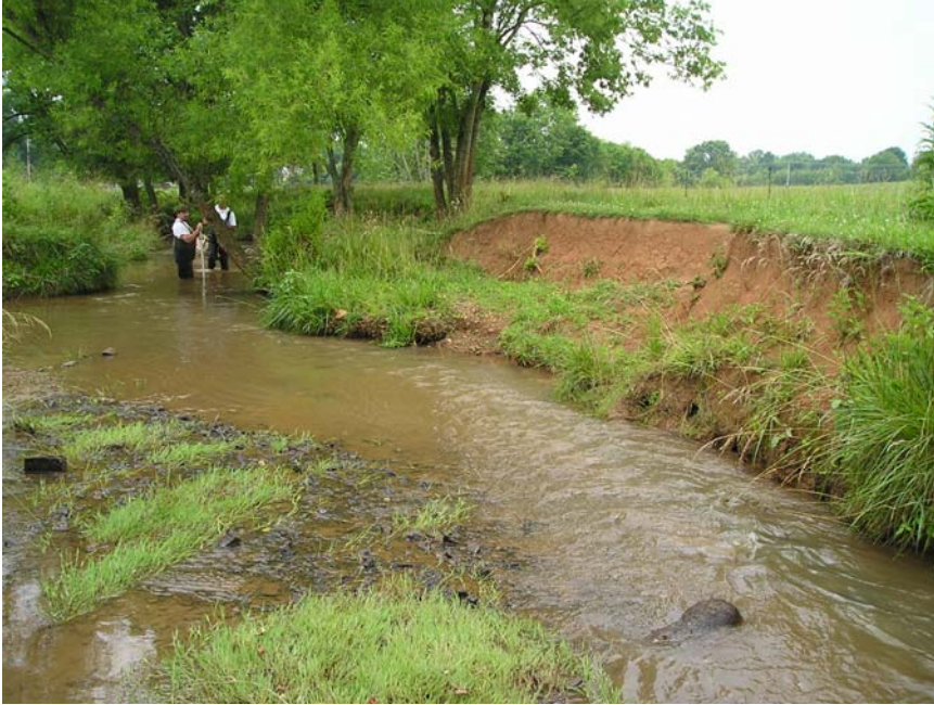
Figure 5: Mass Failure Due to Insision, Site Number STEEK000.7LO
