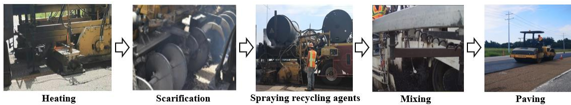
Figure 5-1. Hot in-place recycling procedures.
