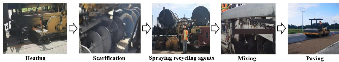
Figure 2-1. Hot in-place recycling procedures.
