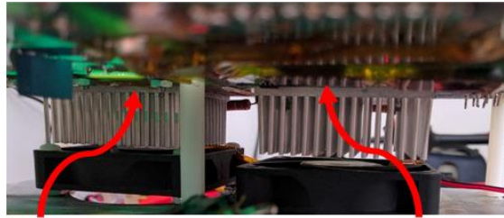
Fig. 5-96. Heatsink and fan installation for the two-stage charger.
