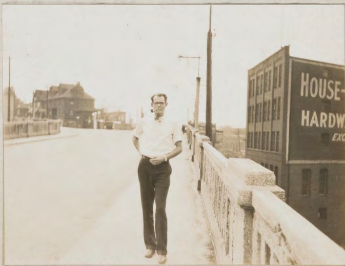
Western Avenue Viaduct above Project No. 2.
