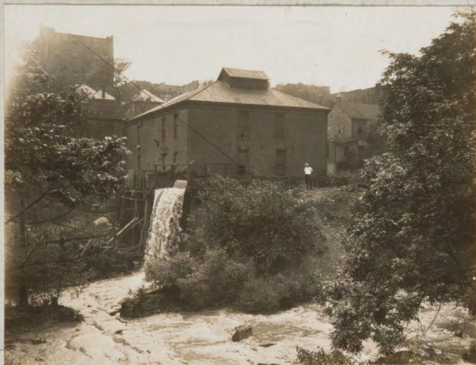
Henderson Milling Co adjacent to location for Project No. 1.
