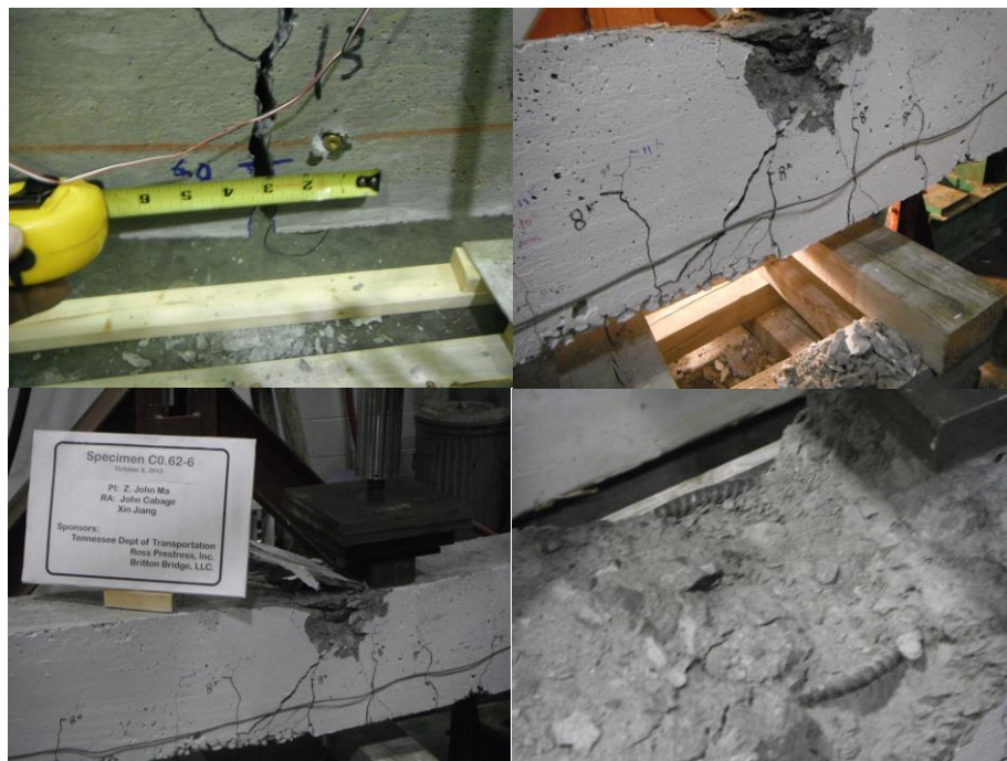
Figure 3.15 – Crack Pattern Collage after Testing
