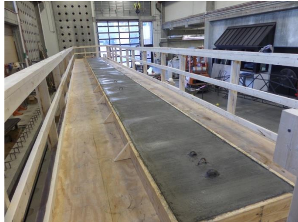
Figure 4.9 – Completed Deck Pour
