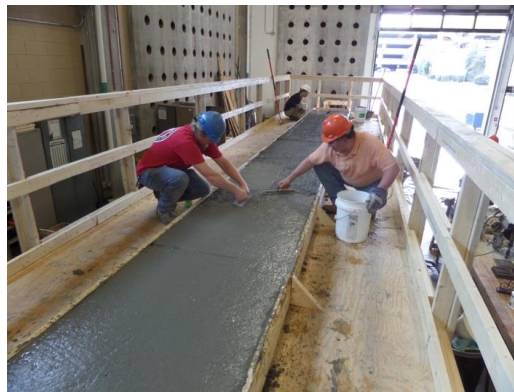
Figure 4.7 – Concrete Deck Finishing
