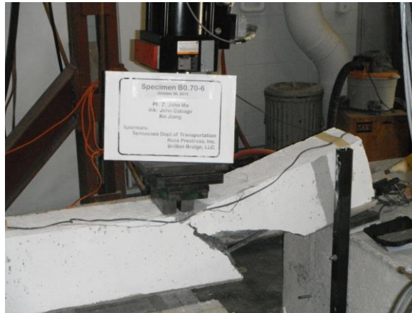
Figure 3.19 – Failure Cracking of Specimen B0.70-6 at Load Point
