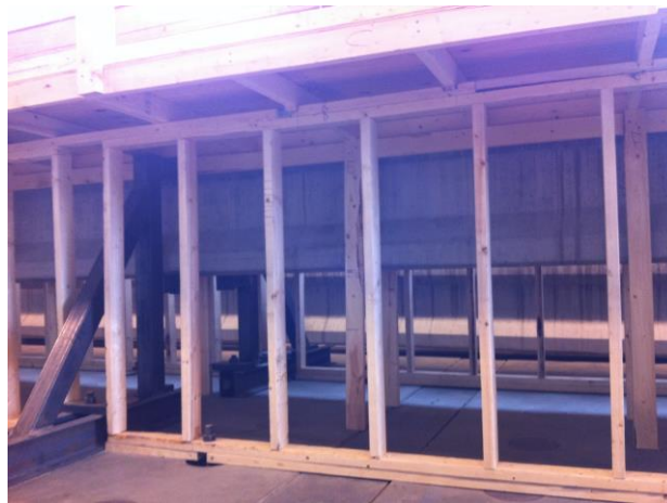
Figure 4.3 – Construction of Formwork Support Structure Showing Beam Side Supports
