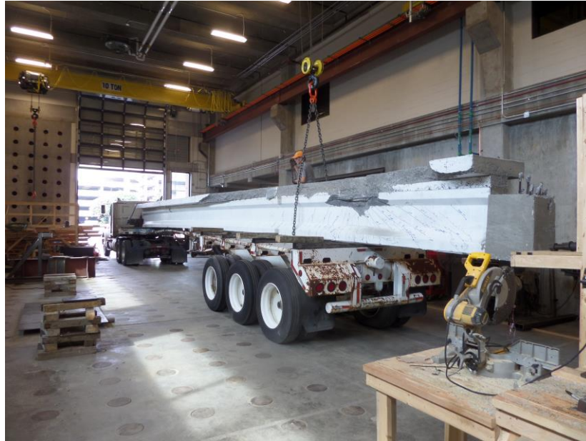
Figure 4.38 – Loading of First Bridge Beam on Truck
