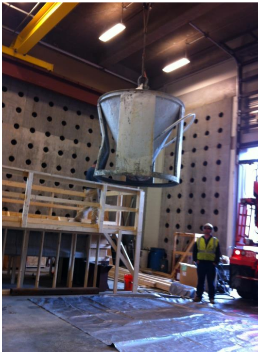
Figure 4.8 – Concrete Placement using a Yard Bucket
