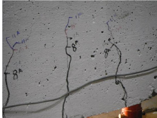
Figure 3.14 – Labeling of Crack Patterns during Testing
