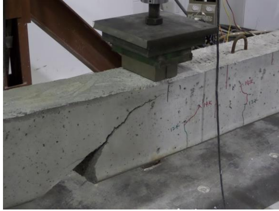
Figure 3.59 – Failure Mode of Specimen B0.62-10
