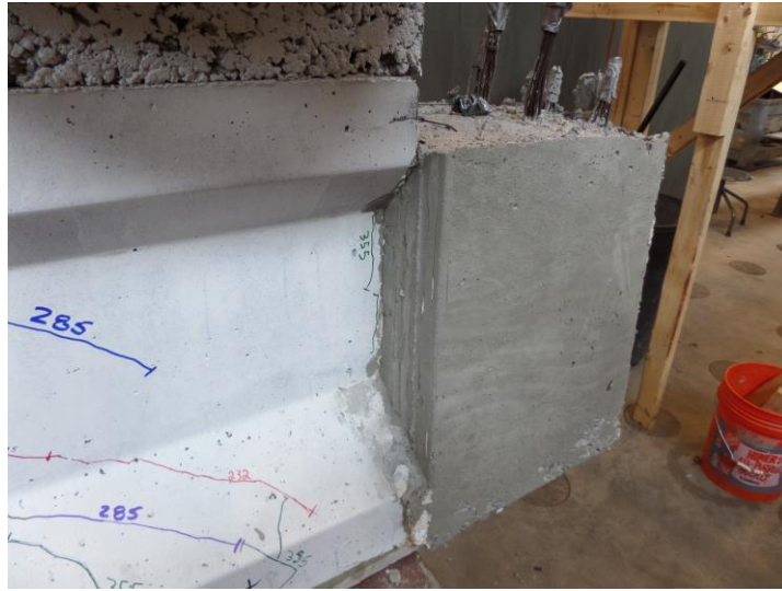
Figure 4.33 – Crack Formed by Rotation of End Block
