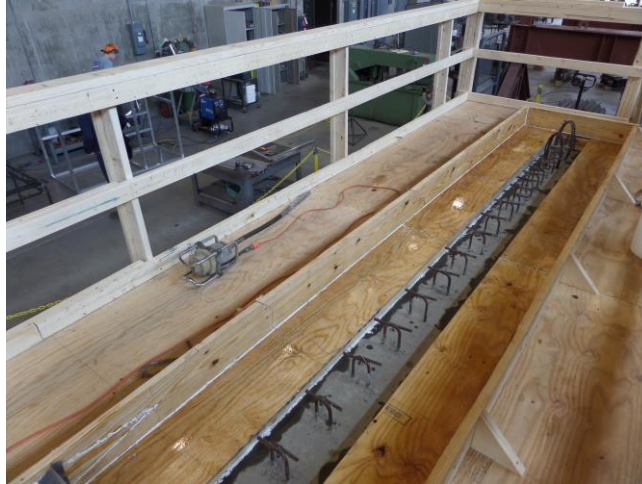
Figure 4.5 – Handrails, Composite Deck Form Boards, and Form Preparation
