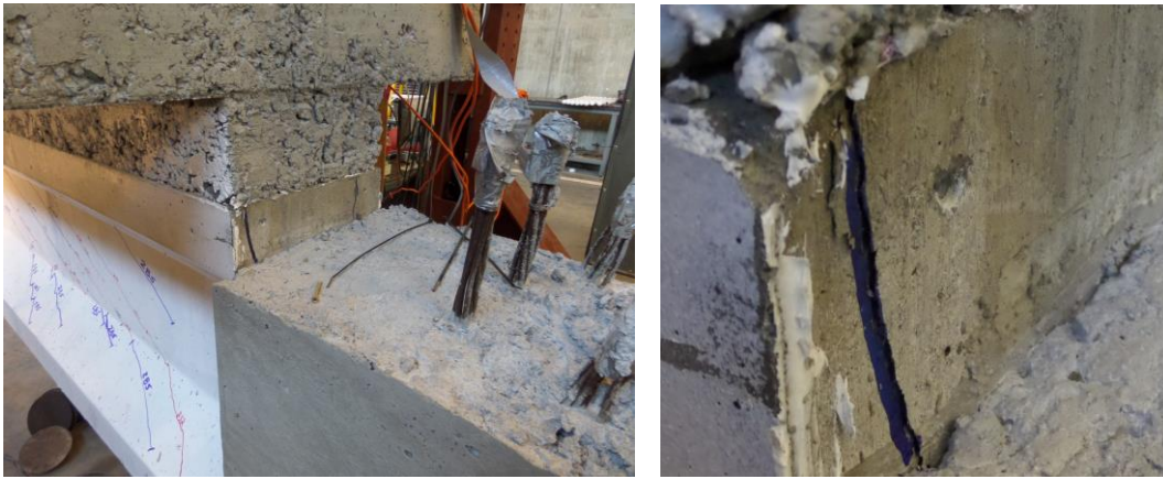
Figure 4.35 – Vertical Top Flange Cracks, Specimen 0.70B
