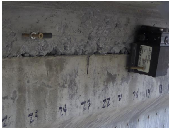
Figure 4.13 – String Potentiometer used to Measure Horizontal Shear at Deck Interface
