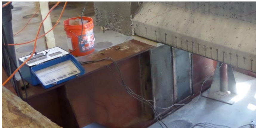
Figure 4.1 – Close-up of Support Modifications
