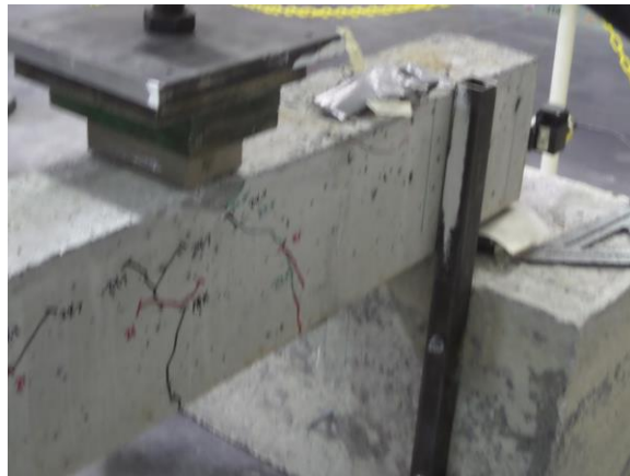
Figure 3.40 – Failure Mode of Specimen B0.70-10
