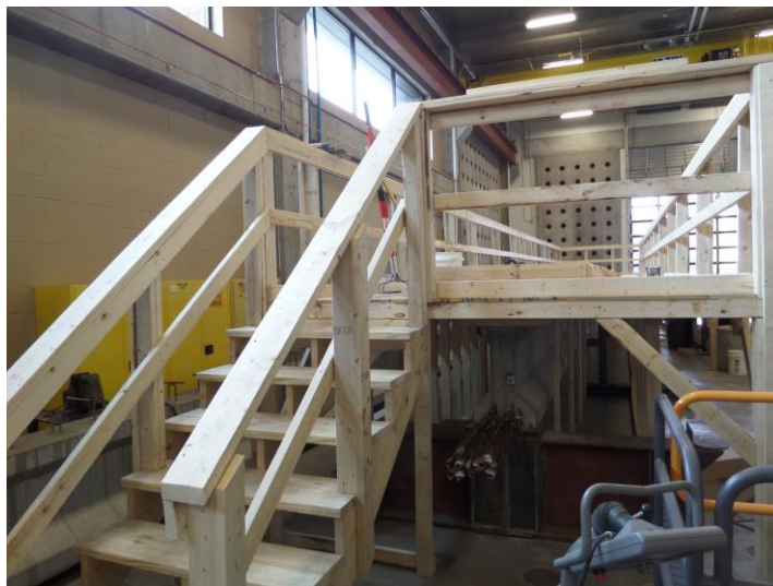
Figure 4.4 – Staircase for Work Access
