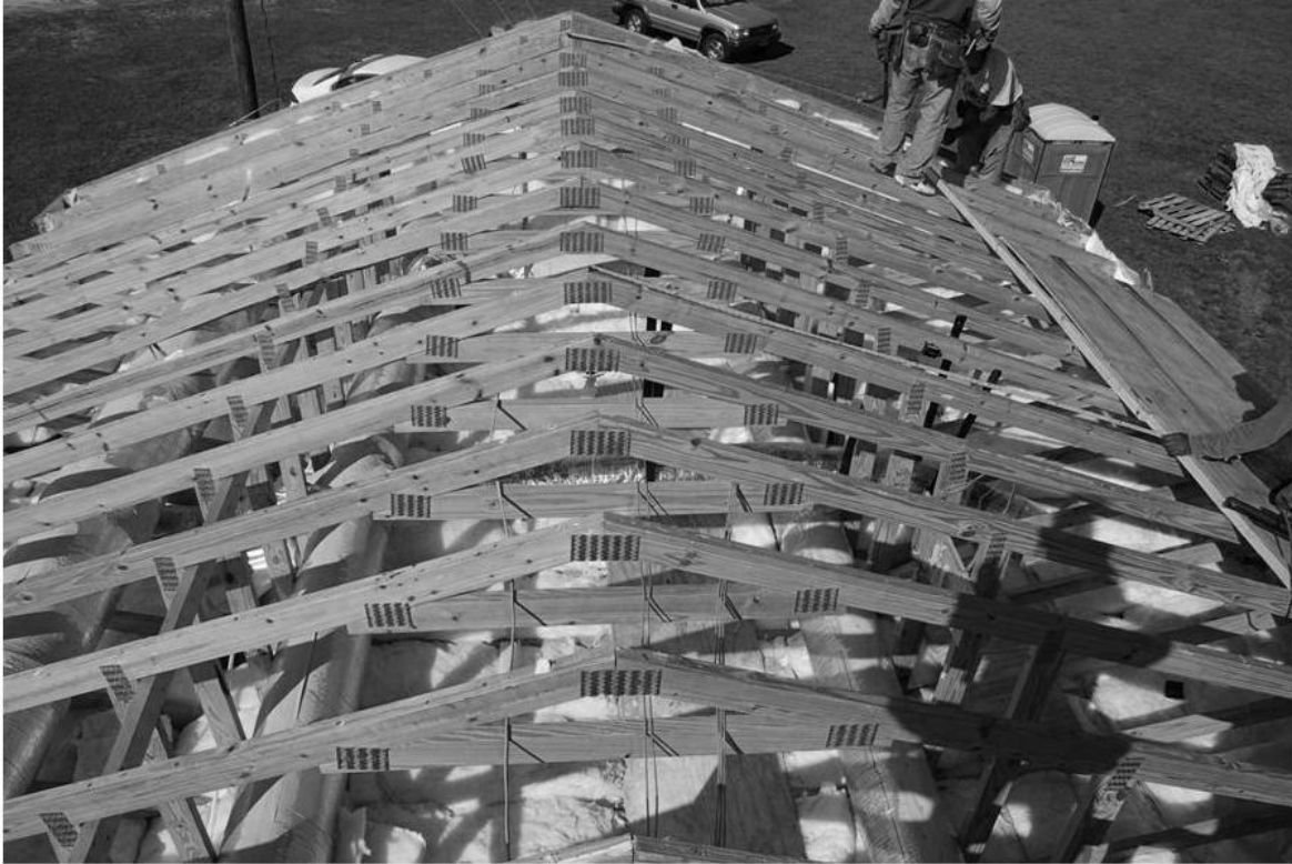
Figure 1: Attic Bay Construction
