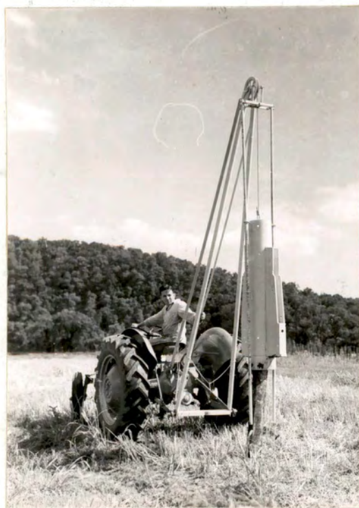
Figure 11 Post Being Driven by Tractor Power
