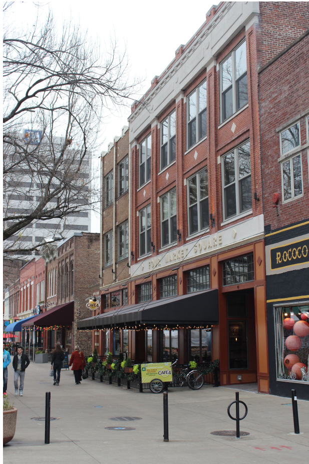
Front view of the building
