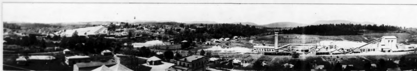
GENERAL VIEW OF AMERICAN ZINC CO. CONCENTRATING PLANTS AND MINE HOUSES, MASCOT, TENN. (ON TENNESSEE RIVER.)
