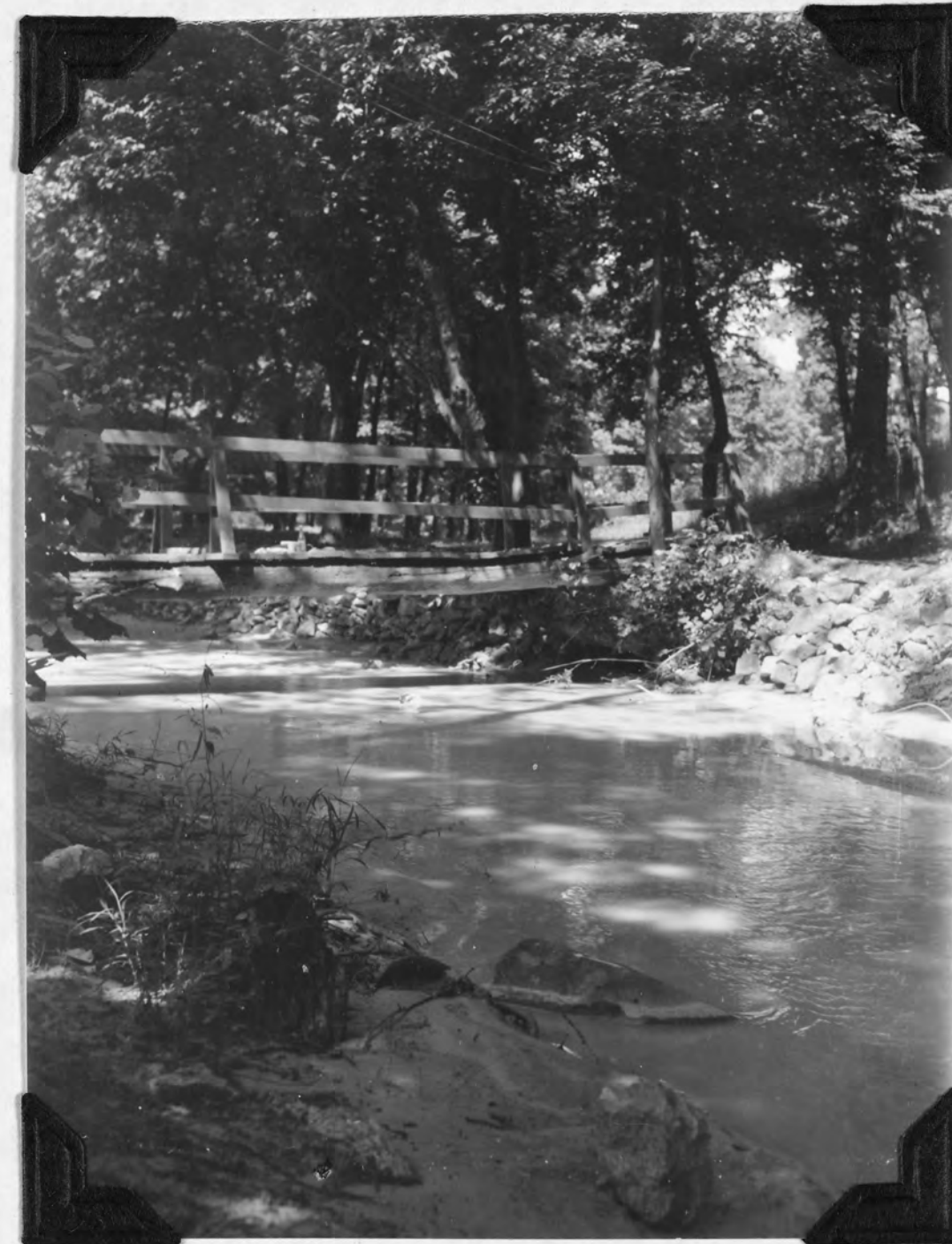
RUSTIC BRIDGE IN TYSON PARK
