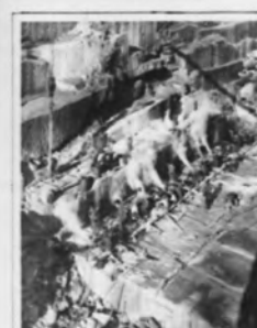
QUARRYING TENNESSEE MARBLE FOR J.P.MORGAN & CO. BANK BLDG. N.Y.
