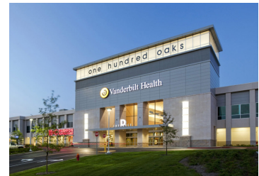
Figure 06. 100 Oaks facade after renovation by Gresham Smith and partners.
