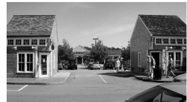
Figure 14. Shallow liner stores at Mashpee Commons.
