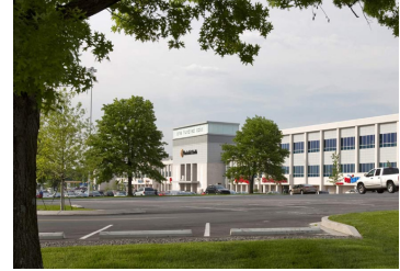
Figure 09. 100 Oaks renovated parking with increased vegetation.
