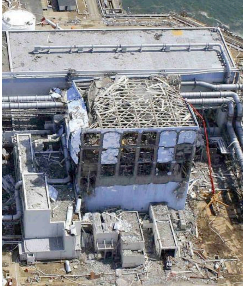
Figure I.1. Building damage caused by hydrogen explosion at Fukushima. Source: Air Photo Service Co. Ltd., Japan
