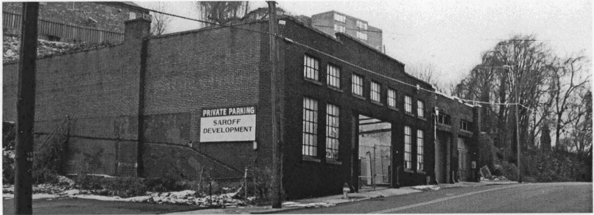
Fig. 6 - 6: Masonry construction source: Author
