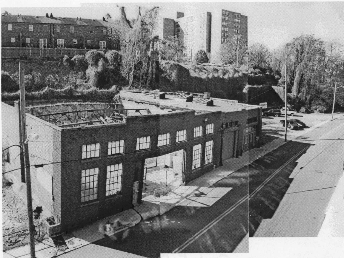
Fig. 6 - 20: Front facade source: Author
