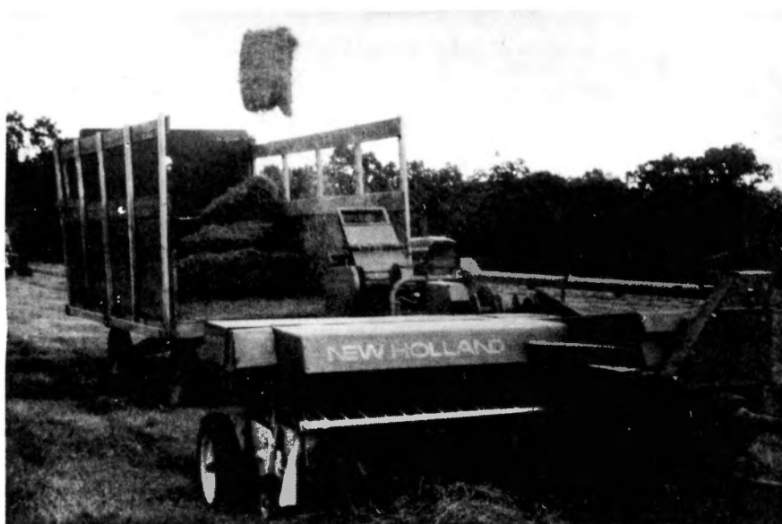
Figure 1. Conventional baler packaging and throwing bales of hay into a trailed wagon.
