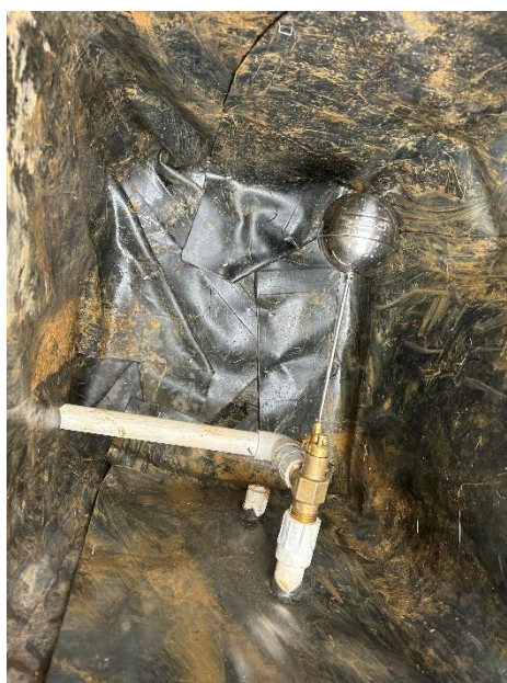
Figure 7: Valve Connection and Waterproof Lining
