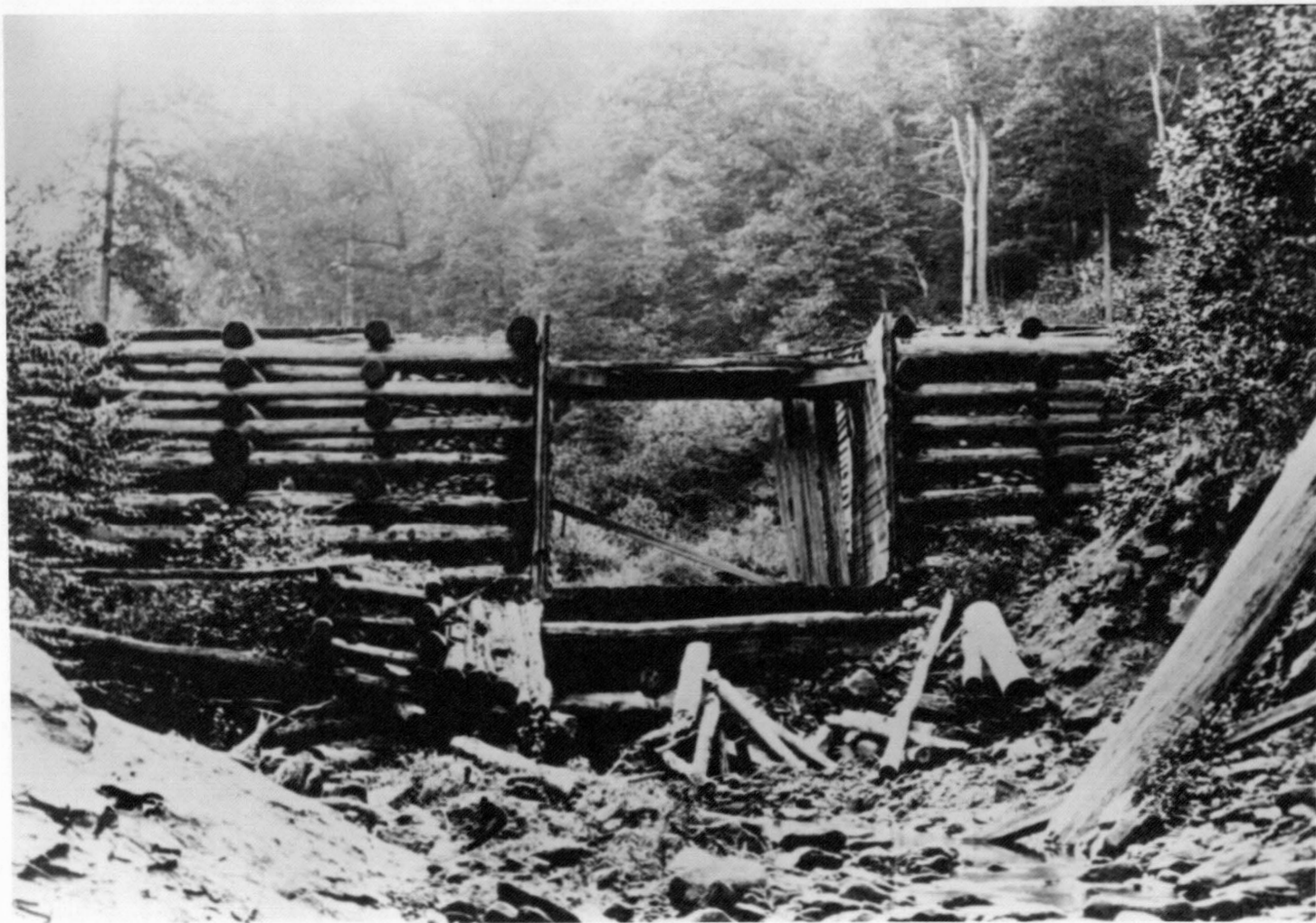
Figure 2. Splash dams were used on streams to develop a water head sufficient for river-driving of sawlogs in the Southern Appalachians.
