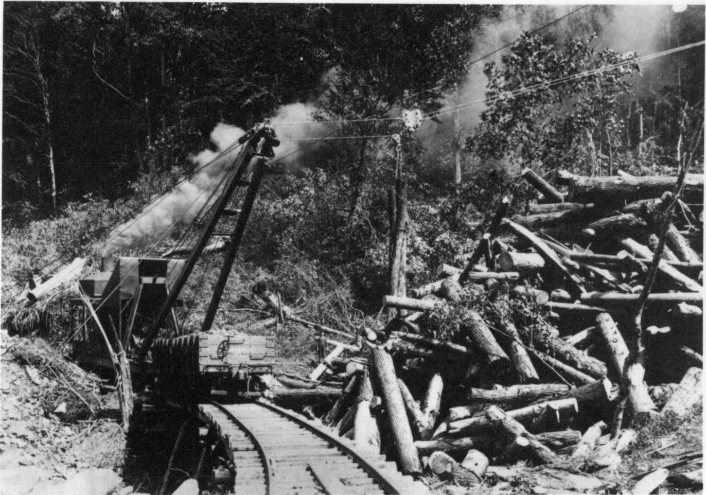
Figure 10. Overhead skidder log landing on Little River showing average log size was between two and a half and three and a half feet in diameter.
