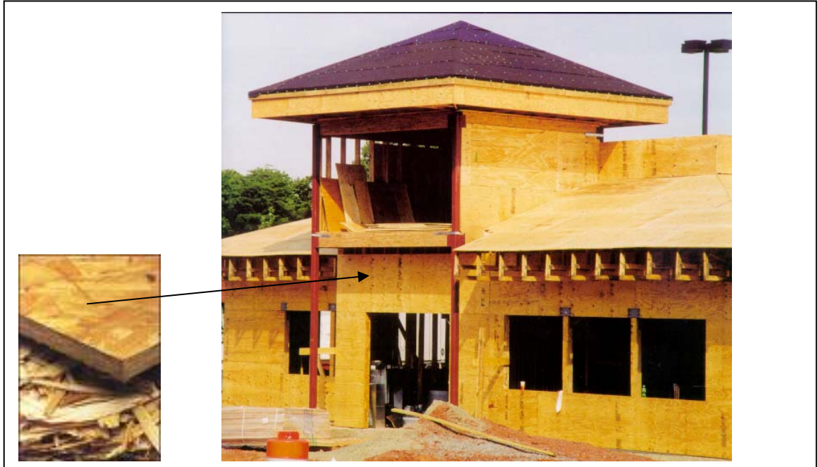
Figure 1. Illustration of OSB wood strands, panels and uses in construction.
