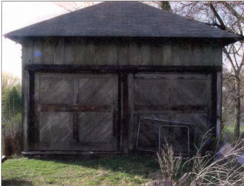
Figure 39. Parks garage, eastern facade.
