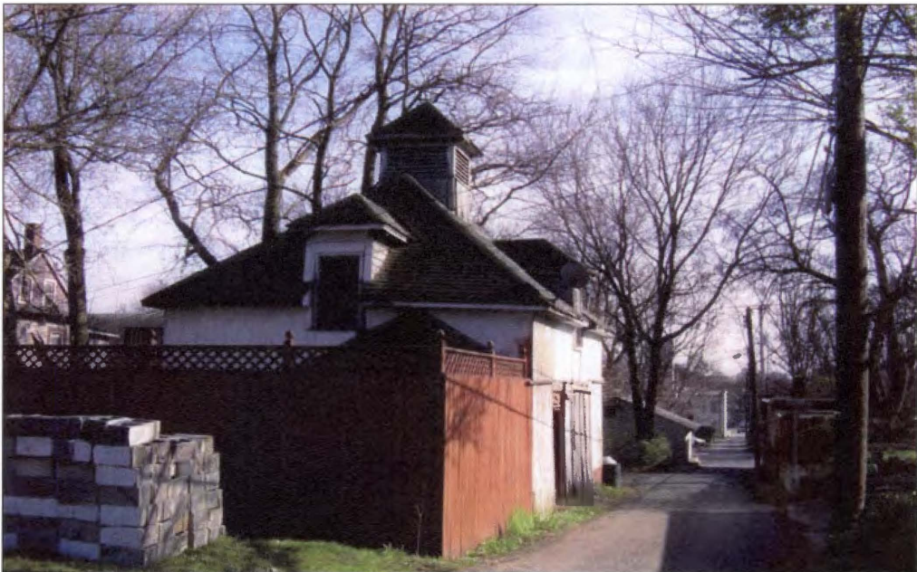
Figure 45. Johnson carriage house, northwest elevation.
