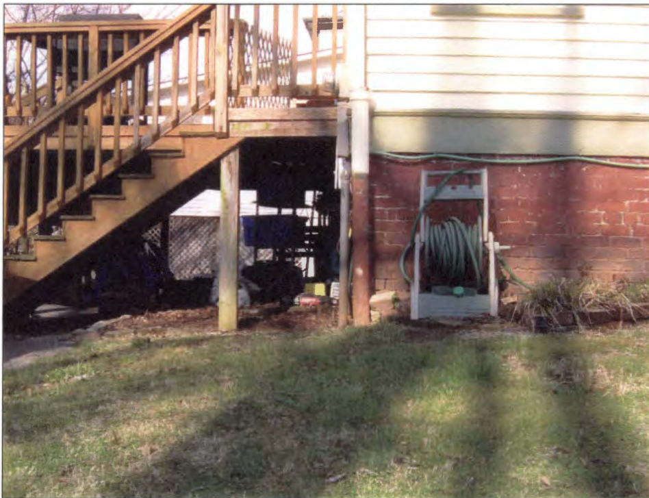
Figure 7. West elevation of the McBrearty house showing the location of the cistern.
