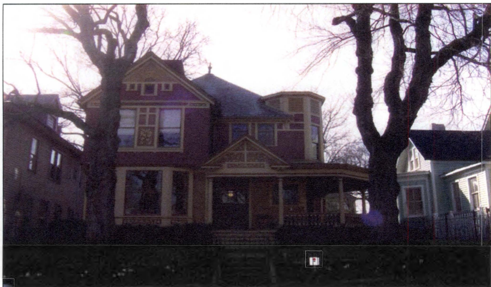
Figure 44. Johnson house, southern facade.
