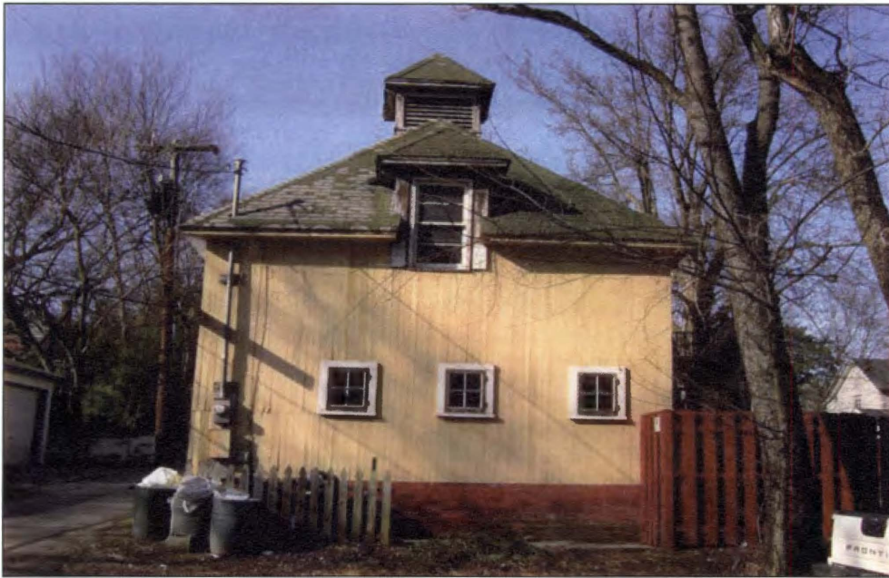
Figure 48. Johnson carriage house, southern elevation.
