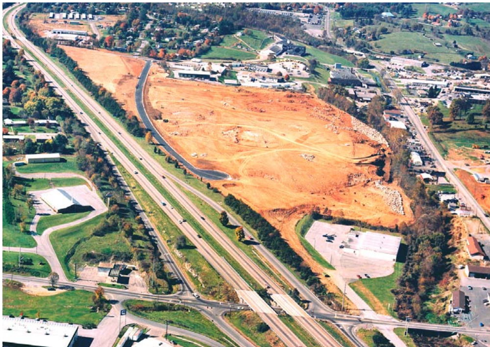
Figure 16: Exit 7 during development(1996). Source: City of Bristol, Virginia.
