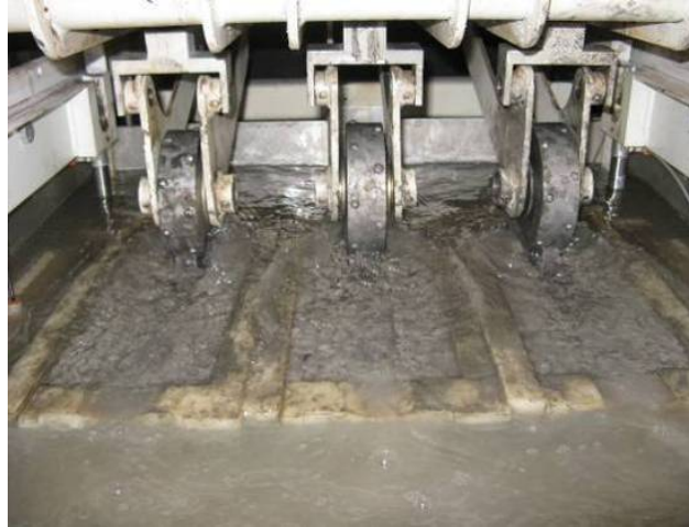
(b) Water submerged condition
