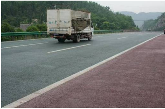
(a) Immediately after construction
