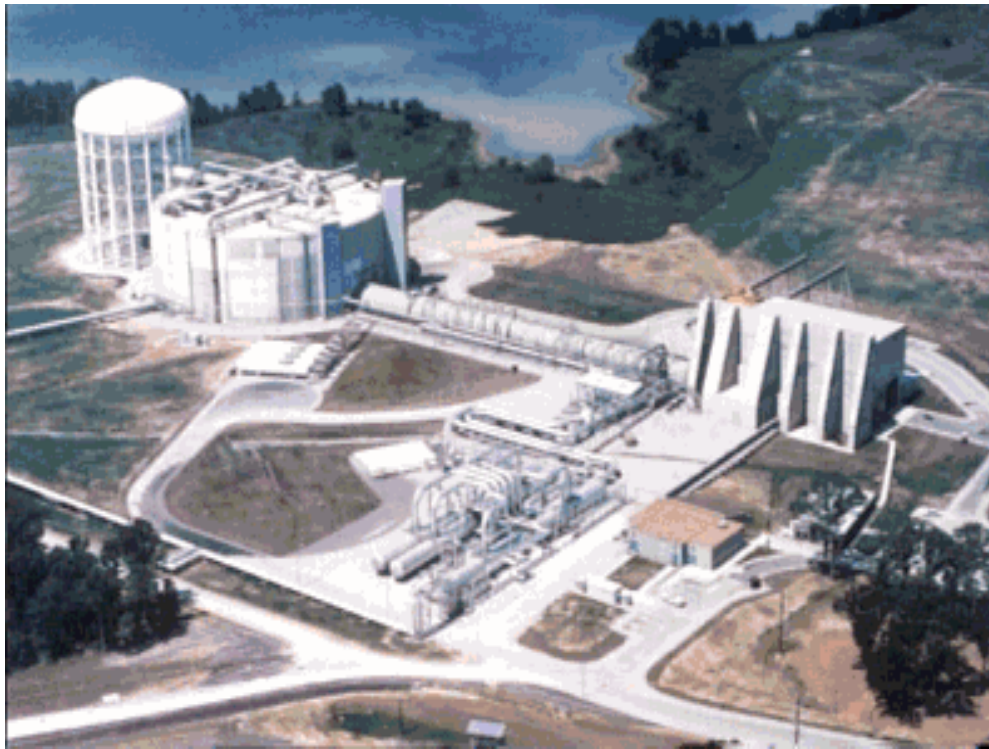
Figure 1. Arnold Engineering Development Complex's J-6 Rocket Test Facility [4]
