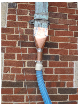
Figure 20 – Downspout adapter. This piece was handcrafted by one of the Facility Services employees that helped with the construction of the RHS.
