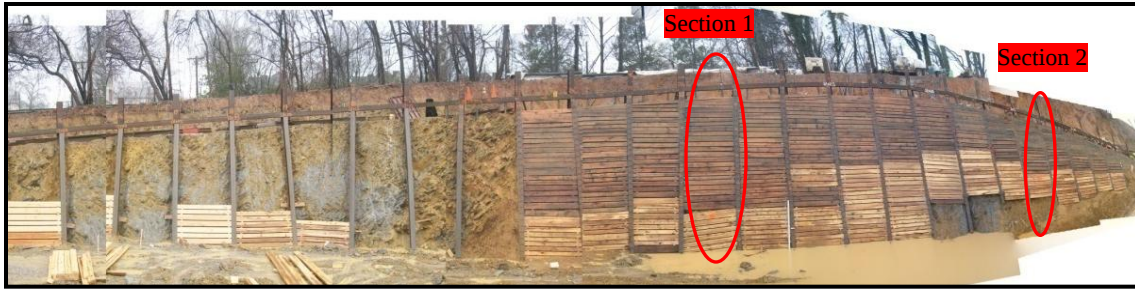
Figure 1-4. Soil Profile of Excavated Wall
