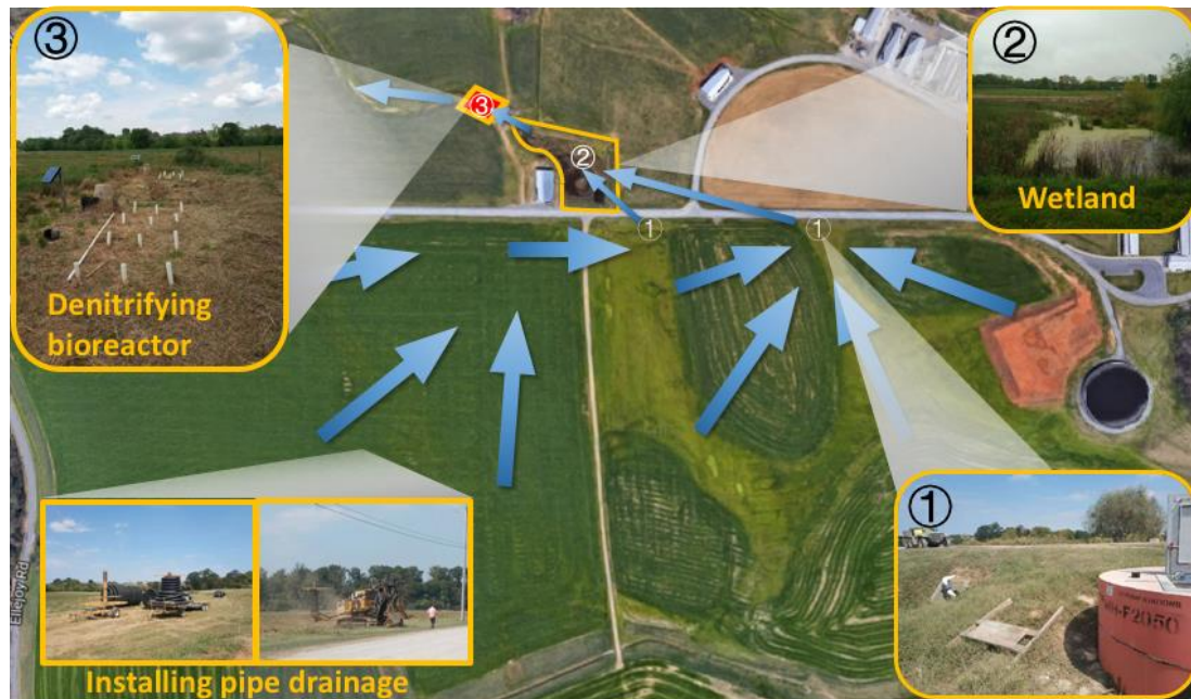
Figure 5.1 An aerial view of the East Tennessee AgResearch and Education Center (ETREC) at Little River Animal and Environmental Unit (LRAEU), red circle is the bioreactor location (Source: Google maps). At the LRAEU, Knoxville, TN the climate is hot and humid with an average summer temperature of 25°C (19 °C -31°C) and average winter temperature of 6°C (0°C- 11°C). (1) is the drainage station; (2) is the wetland which details can be seen in Fig 16; (3) is the field denitrifying bioreactors.
