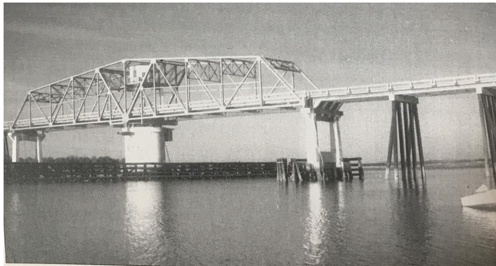
Figure 3: The first bridge to Hilton Head was a drawbridge (Harvey, 1998)
