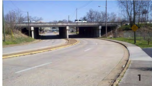
Benard Ave had some existing sidewalks
