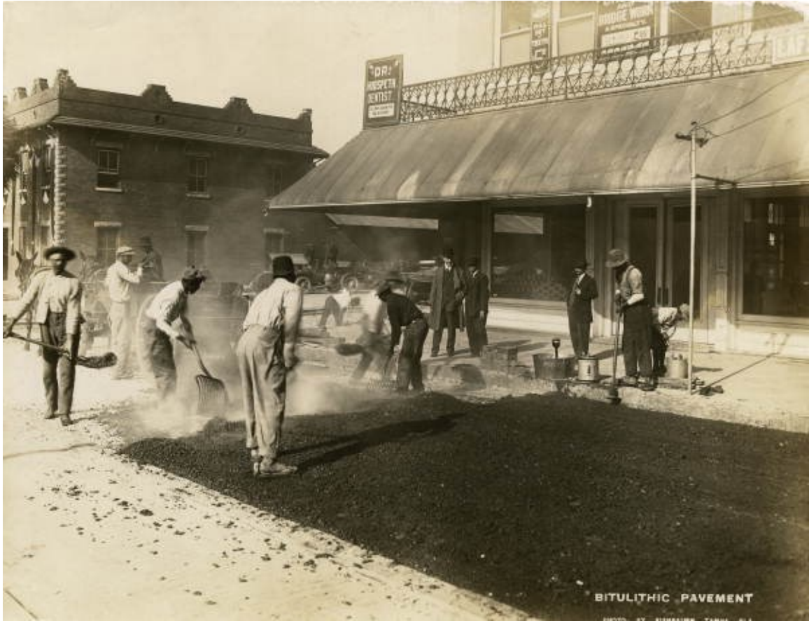
Figure 2.1. Bitulithic pavement placement process. Tampa, Florida (1920s.)
