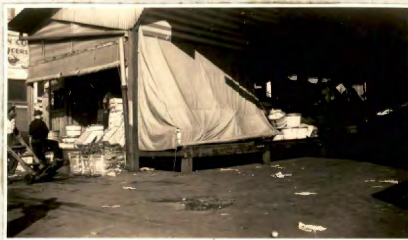
Permanent stall in Trucker Shed No. 2. Space is partially enclosed by canvas. Notice wooden platform 18" off floor, sufficiently high to permit cleaning underneath.
