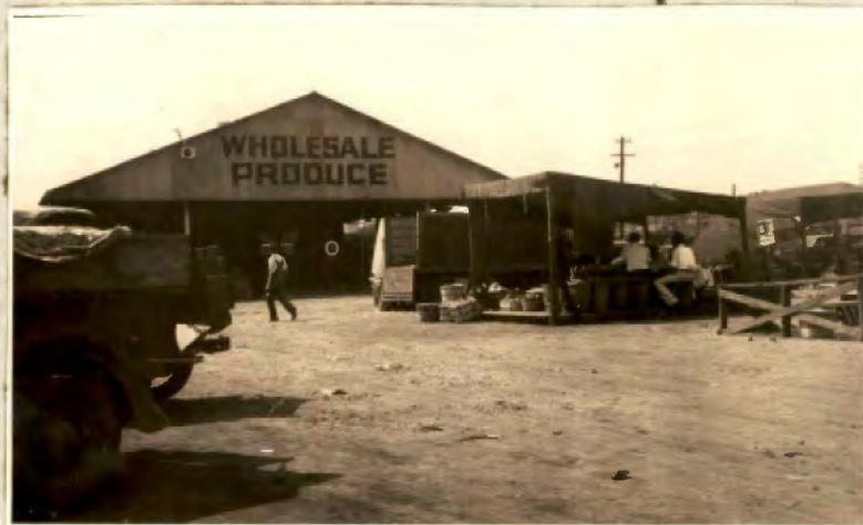
End view of shed, 50 feet wide. Canvas shelter on center right stall.
