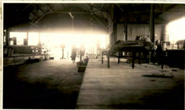
Interior of Truckers' Shed, East End. Platform 2 feet high. Steps are required. Stall units may be walled in with sheet iron as shown on right. Notice arrangement of lights directly over edge of platform.
