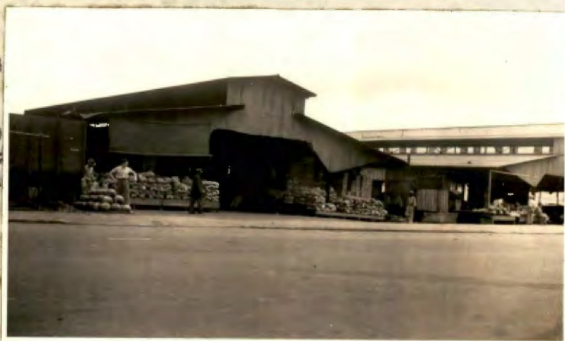
Trucker sheds Nos. 2 and 3 facing Courtland Street. Width from eaves to eaves 60 ft., center driveway 20 ft. Occupied by permanent stallmen. Citrus is piled up on front platforms.
