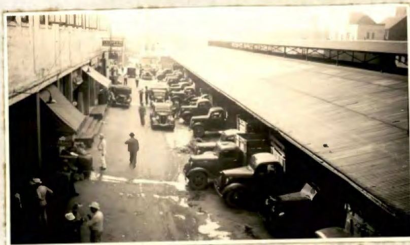
View of "green shed" section of Truckers Shed No. 1 on right. Trucks are not permitted to remain after unloaded. No permanent stalls allowed on this side. Dealer stores on left. Picture taken from Washington Street viaduct.
