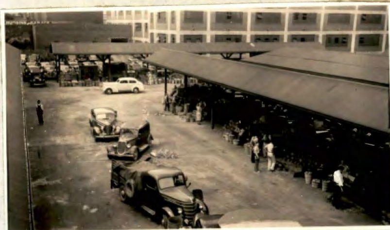
Trucker Shed No. 4 on extreme right, Nos. 5 and 6 on right, and No. 8 in rear center. 40-foot driveway. These sheds are known as "Chinatown", used by out-of-state truckers.
