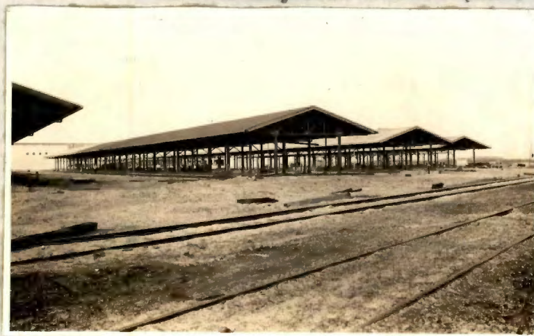
Figure 50. Kansas City Food Terminal (under construction, Sept. 4, 1939).
