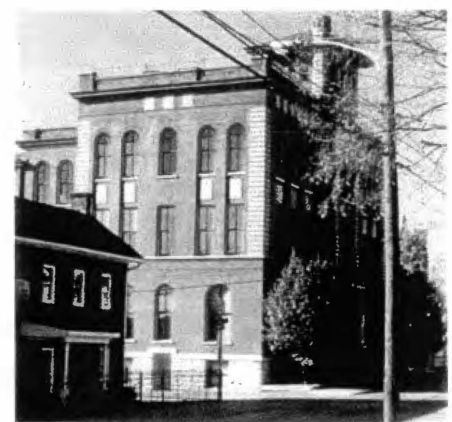
Figure 3. 5: Renovated Vanderbilt University building
