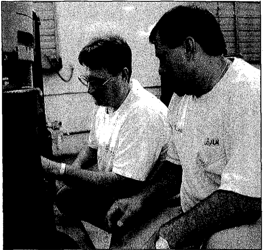
Steve Wyatt, MTAS utility consultant, and Vincent Hurst, maintenance technician, rewire control circuits at a Jackson Utility District water plant.
