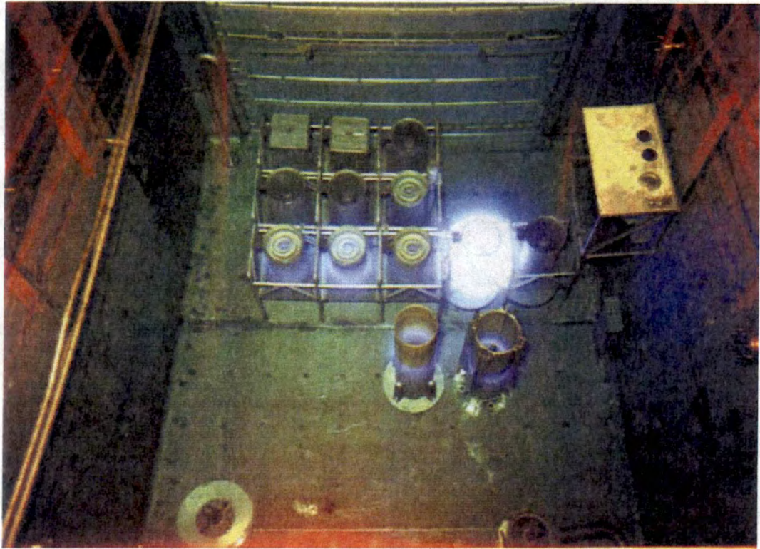
Fig. 3.7. SNF elements in the HFIR SNF pool.
