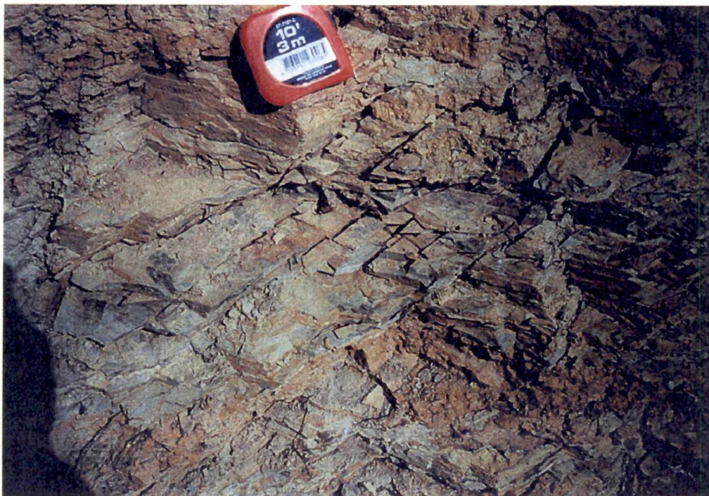
Typical array of fracturing, photograph is mostly shale saprolite.
