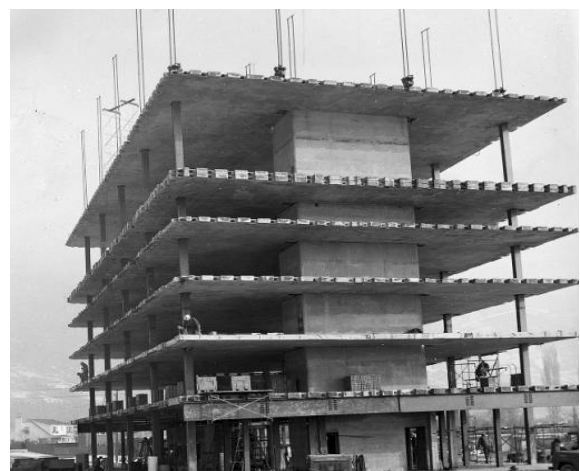
Figure 11: Lift slab construction technique
