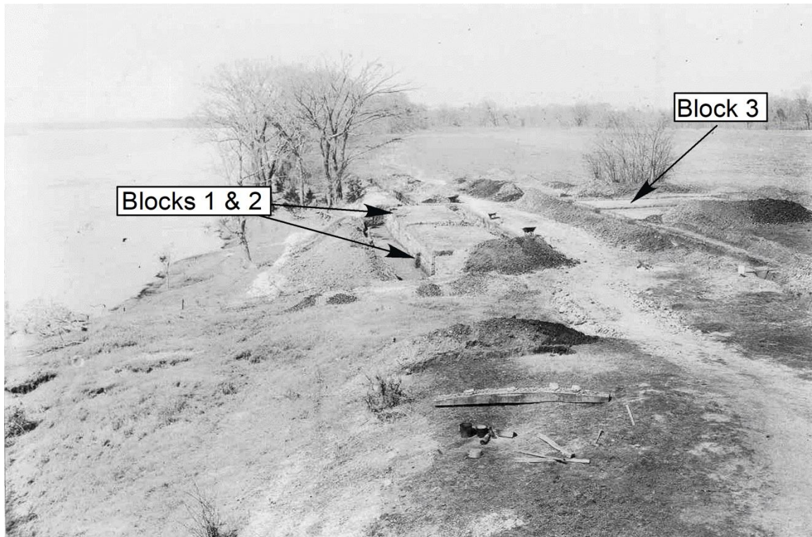
Figure 7.3. View to the west of the Whitesburg Bridge site in the Winter of 1939 (photo courtesy of the Alabama Museum of Natural History).
