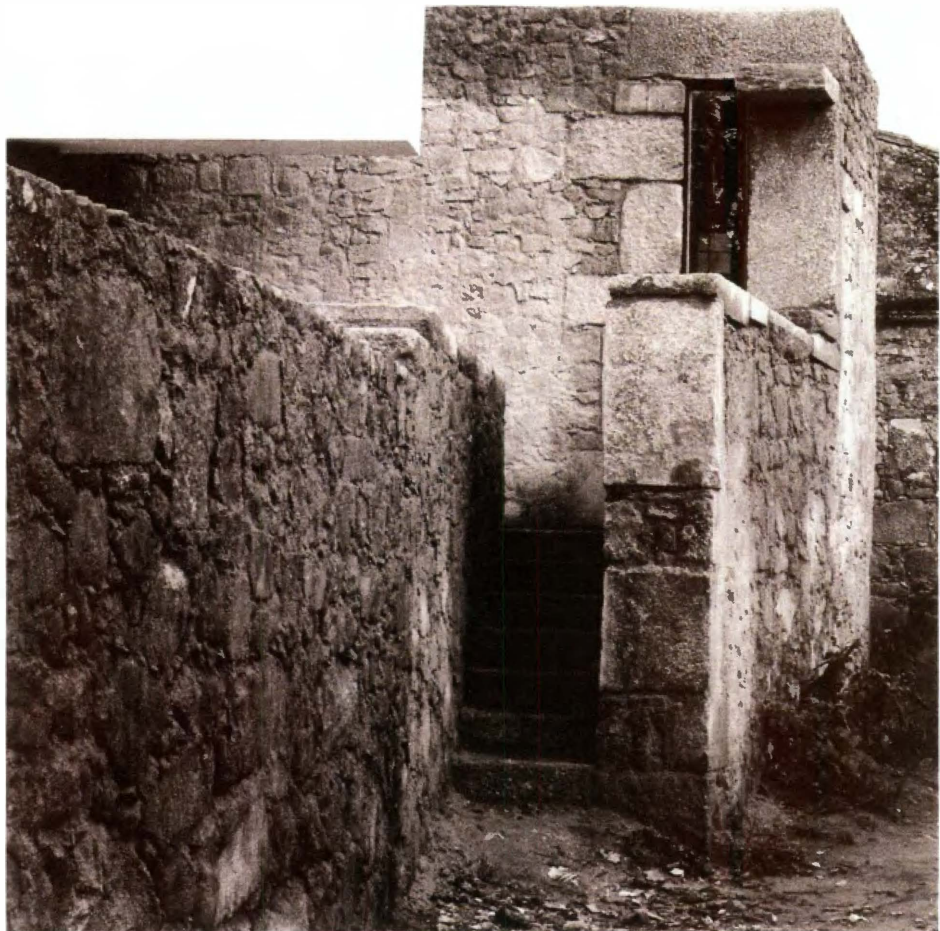
Fig. 6B-4 View of existing structures on building site (Esposito)
