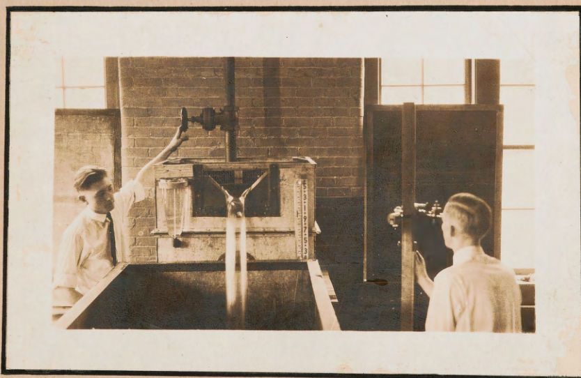
A FRONT VIEW OF THE WEIR-TANK SHOWING THE LOCATION AND ARRANGEMENT OF THE RELATED APPARATUS
