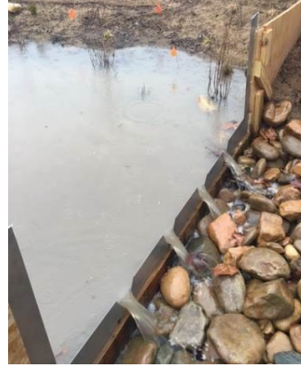
Figure 4.2a-b a) Compound weir located at a) pipe outlet/RSC inlet b) RSC outlet to Baker Creek. Image taken from Thompson et al. (2018) .
