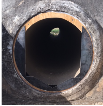
Figure 4.2a-b a) Compound weir located at a) pipe outlet/RSC inlet b) RSC outlet to Baker Creek. Image taken from Thompson et al. (2018) .
