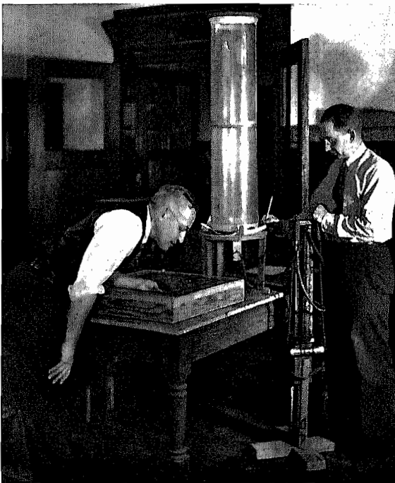
Laboratory apparatus for determining the relative effectiveness of various insecticides on roaches.
