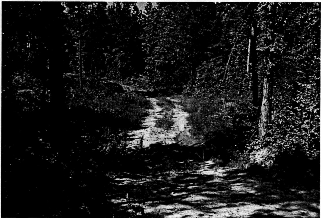
Figure 4. NCAT Pavement Test Track Site Before Clearing and Grubbing, June 1998.
