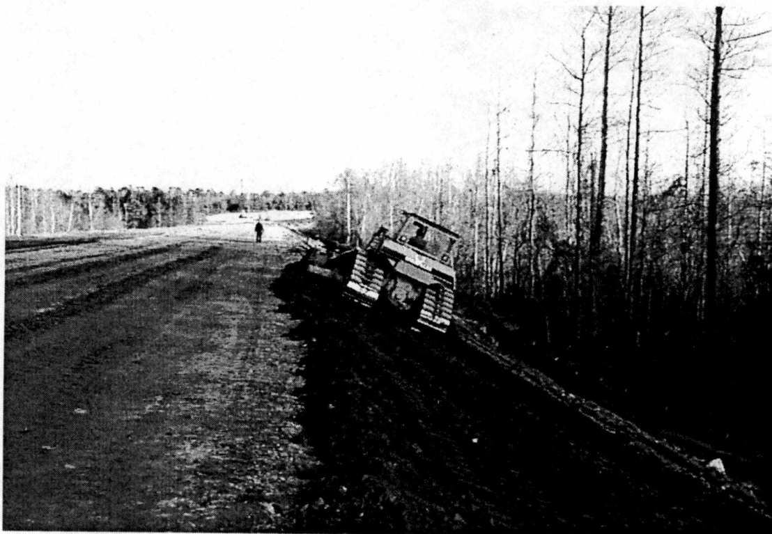
Figure 6. Embankment Placement Along the North Tangent, January 1999.
