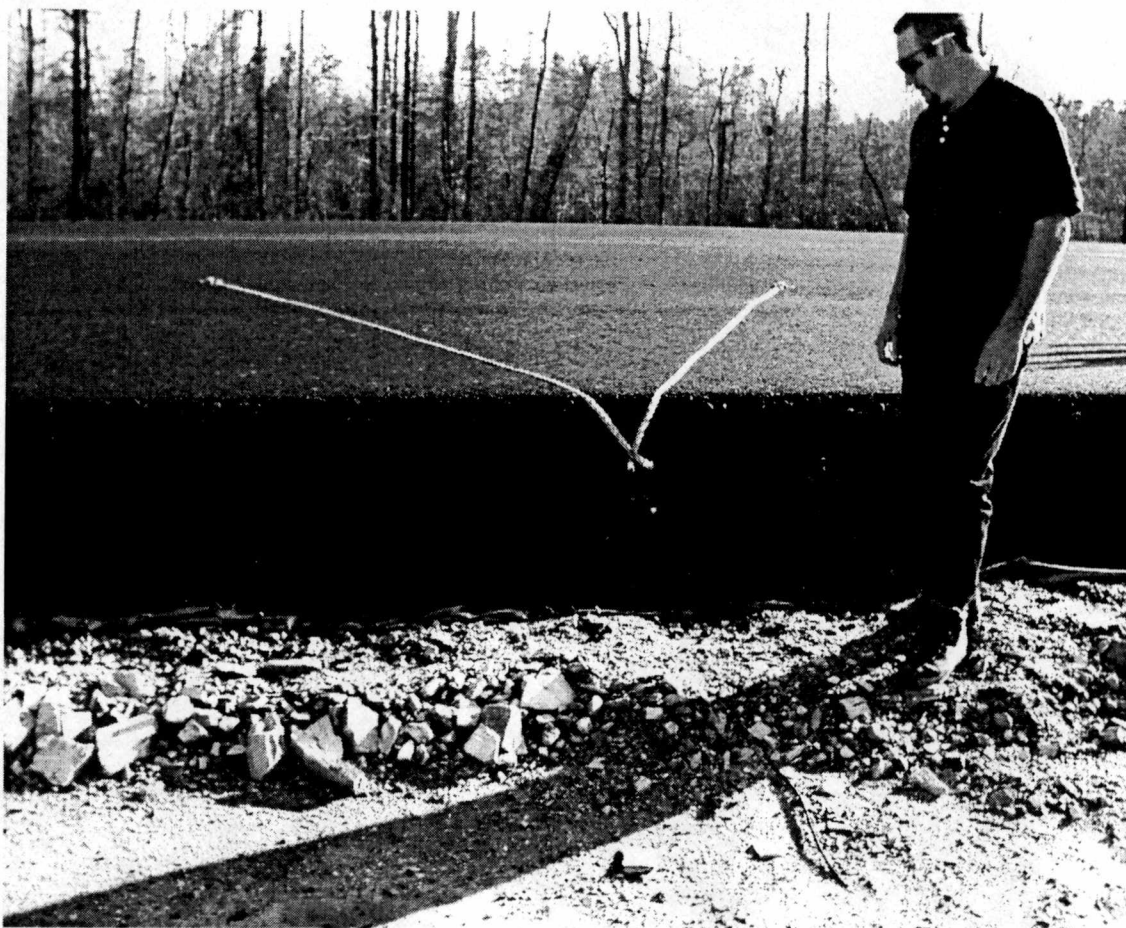
Figure 11. Full Pavement Section up Through the 15 Inches of 37.5 mm Superpave™ Base Course, January 2000.
