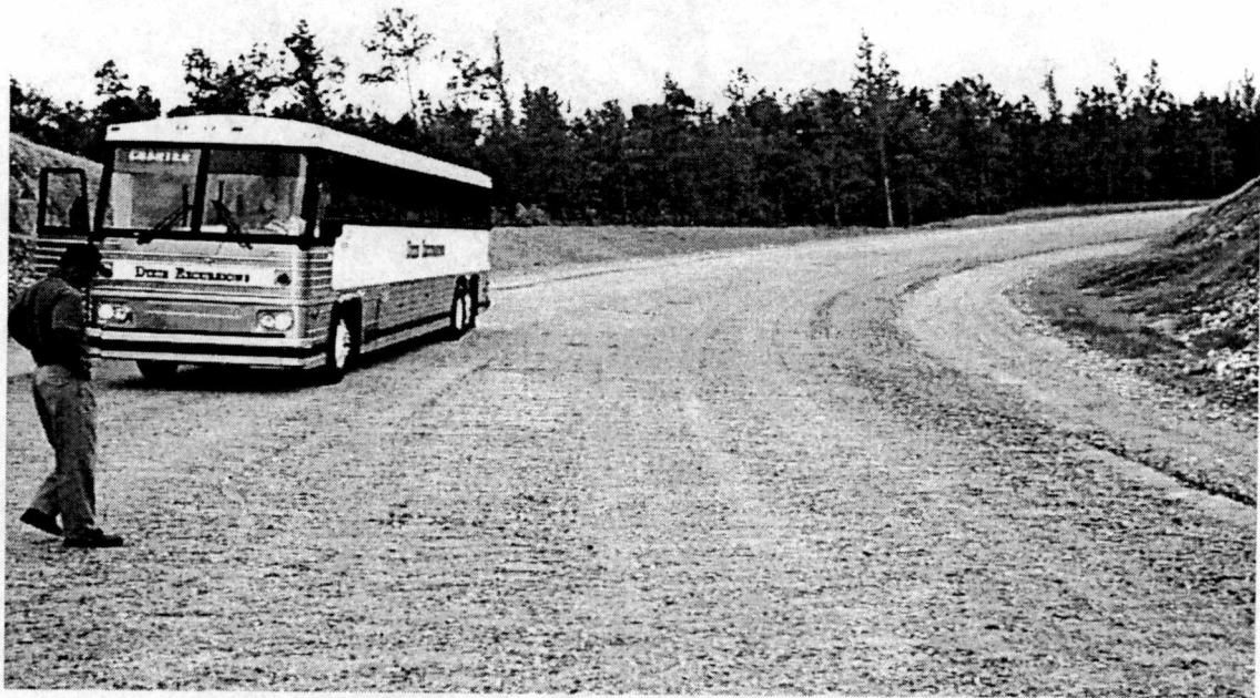
Figure 9. Photo After Placement of 6 Inches of Aggregate Base Course, September 1999.
