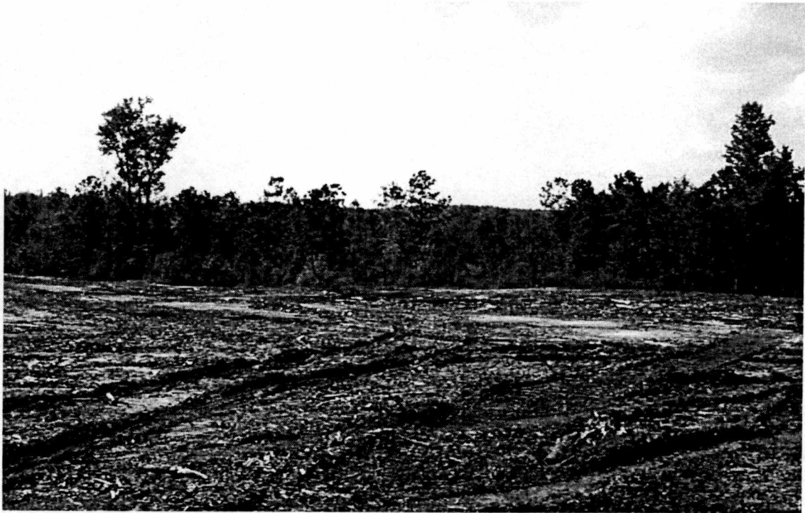
Figure 5. NCAT Pavement Test Track After Clearing and Grubbing, October 1998.
