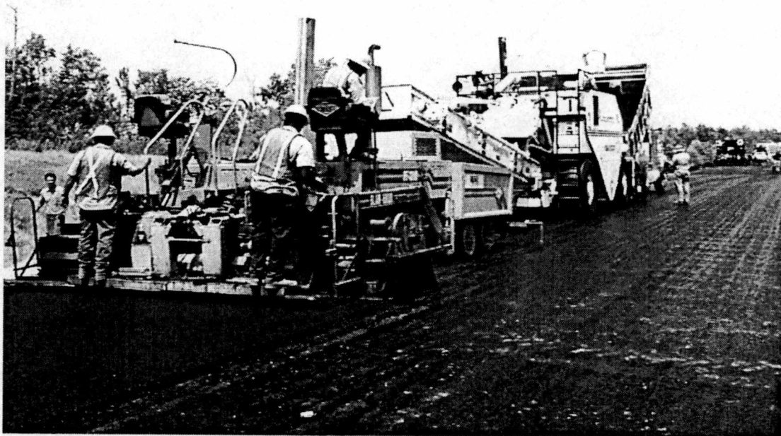
Figure 15. Placement of TDOT Test Section S4 Surface Mix, July 2000.
