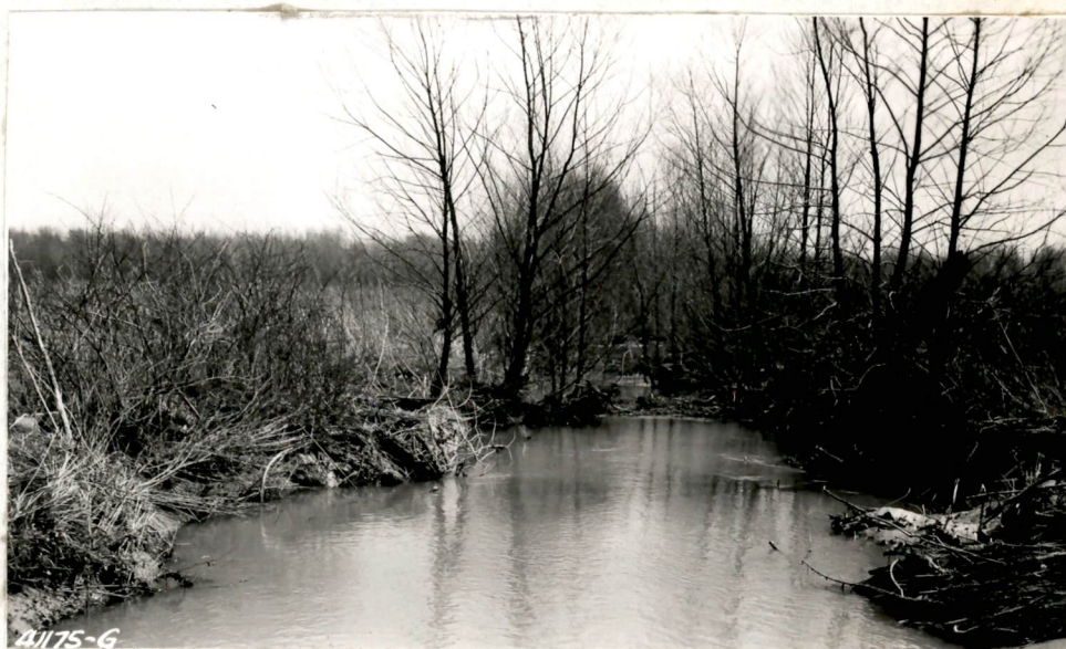
Figure 6. Trees and Drift Hindered Flow in March 1949
