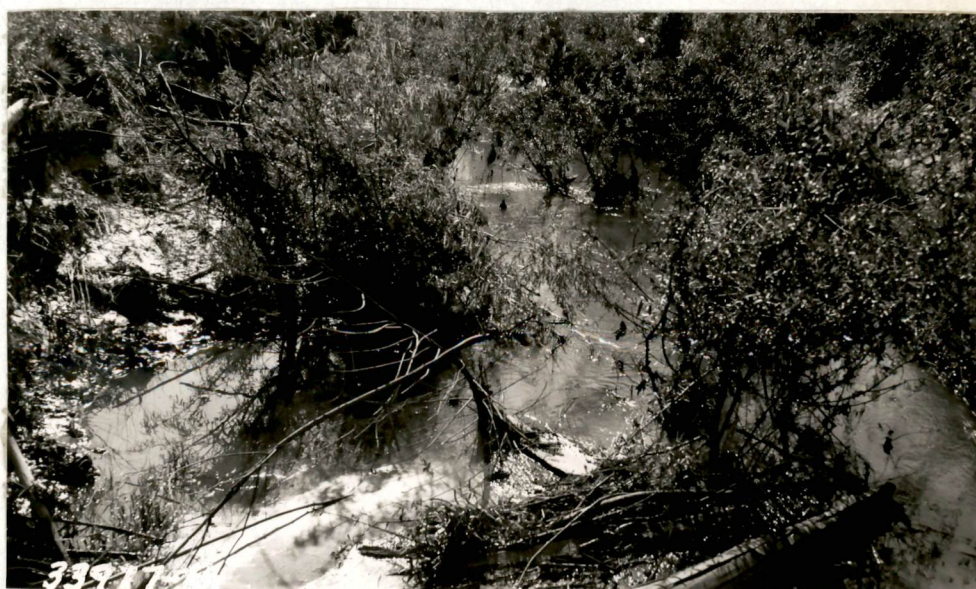
Figure 4. Brush and Debris Above Cane Creek Bridge
