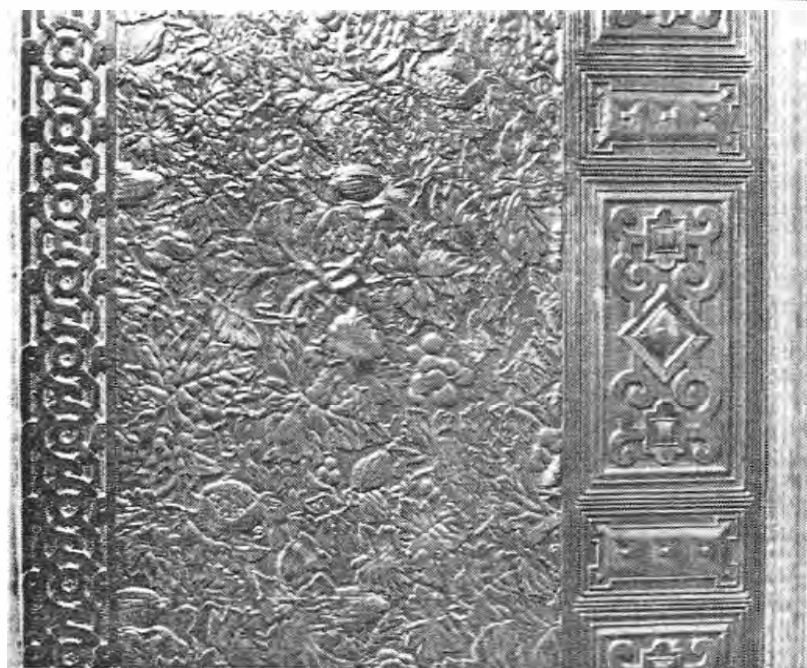
Figure 164. Section and detail of the Lincrusta Walton covering the dado area in the Mallory-Neely dining room.
