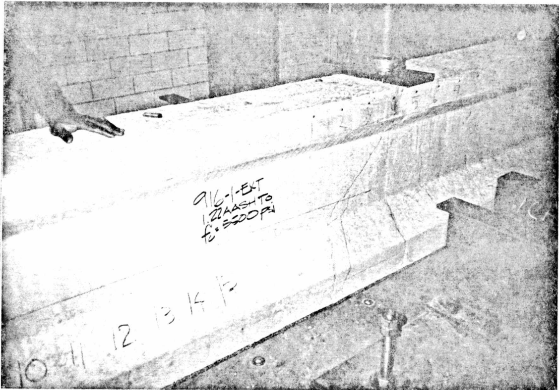
Figure 6.5 Photograph of Flexural-Shear Cracks in Beam 916-1-EXT
