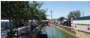
Fig 35 | Canal Cut and Esplanade
