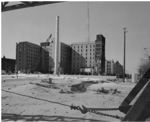
Occidental Hotel and Surrounding Buildings Pre-Demolition
