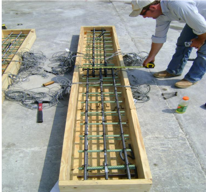
Figure 14: Specimen Construction (a) Reinforcement in the Forms
