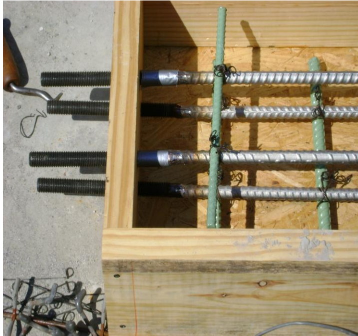
(c) Threaded Rods Extending through the Form
