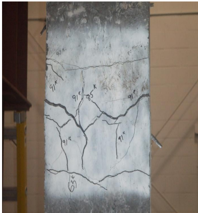
Figure 29: Tension Crack Patterns at Failure (a) Specimen ST-1
