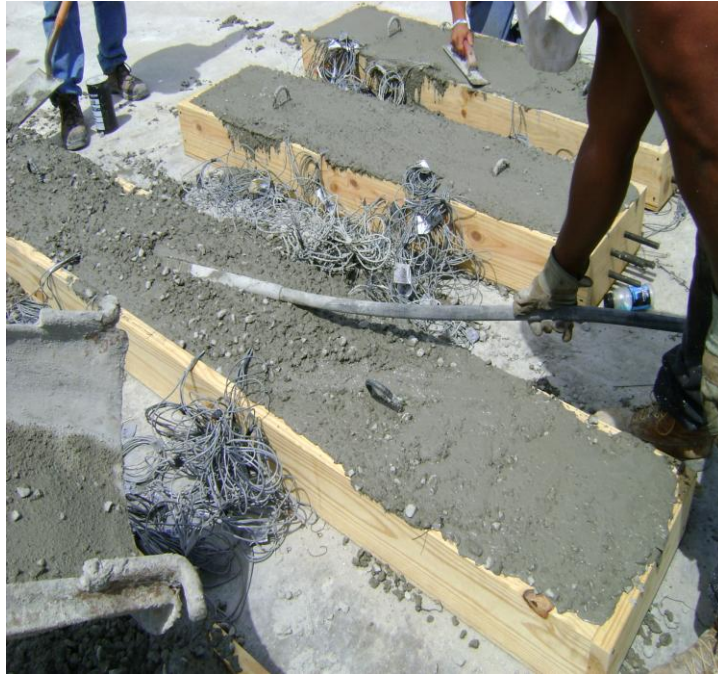
(e) Vibrator Use in the Joint Zone
