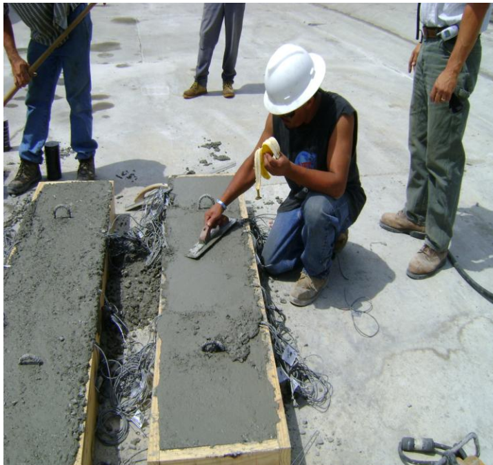
(f) Concrete Finishing
