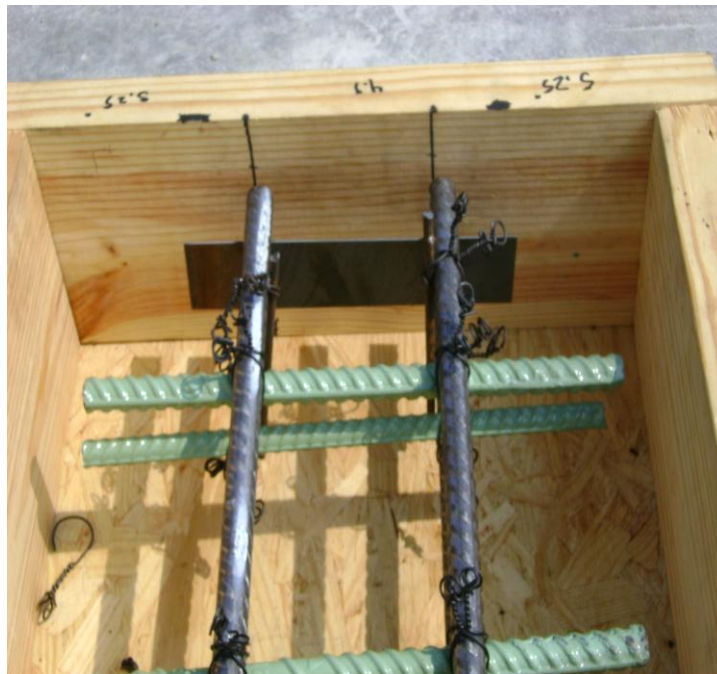
(b) Plate Used to Ensure Proper Layer Separation
