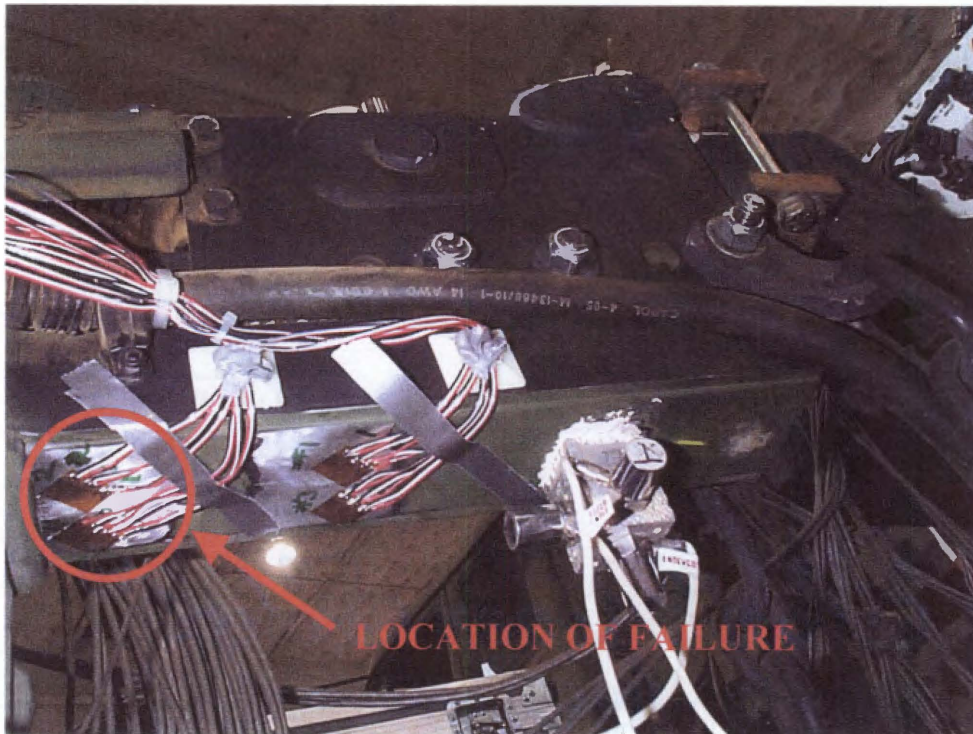
Figure 4.1: Strain gage rosette at failure location.
